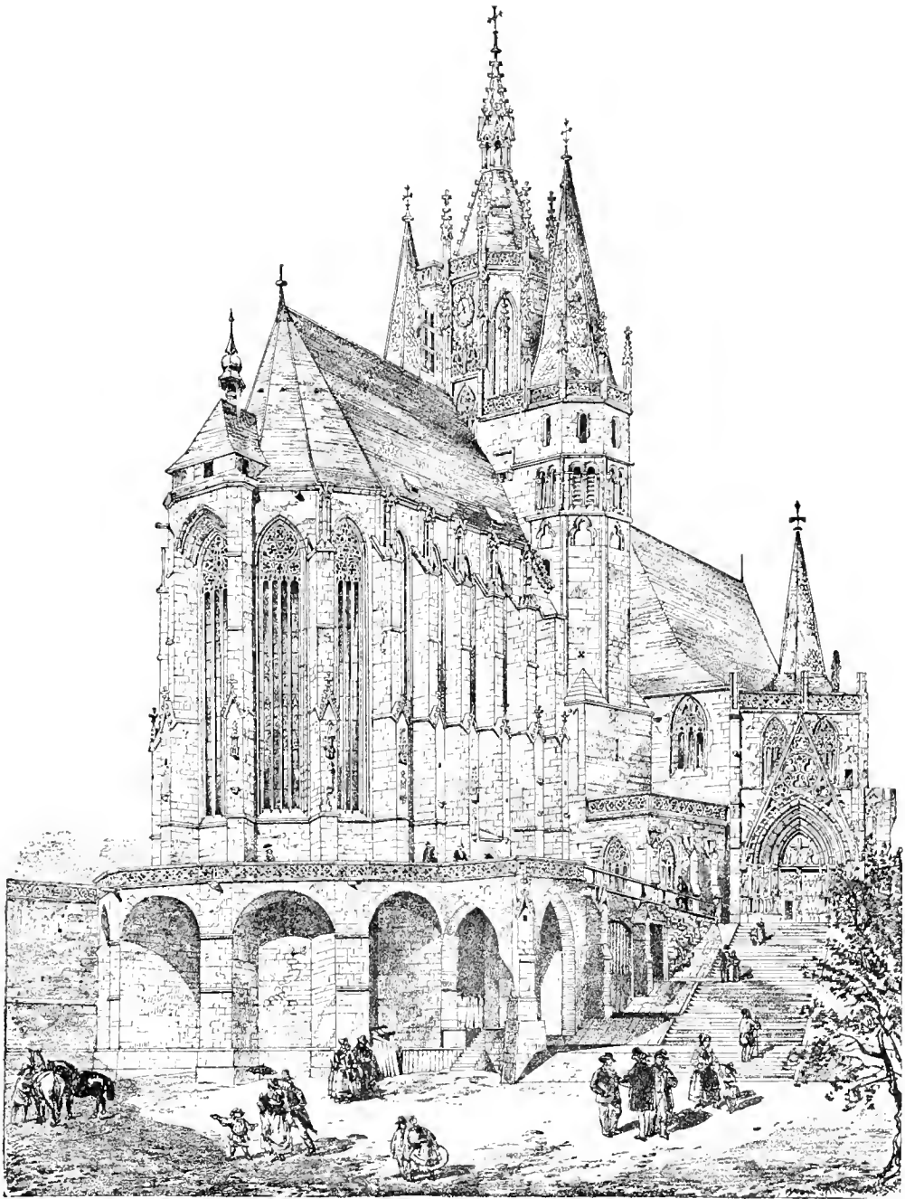
SUBSTRUCTURE OF CHOIR OF CATHEDRAL: ERFURT, SAXONY, GERMANY.
